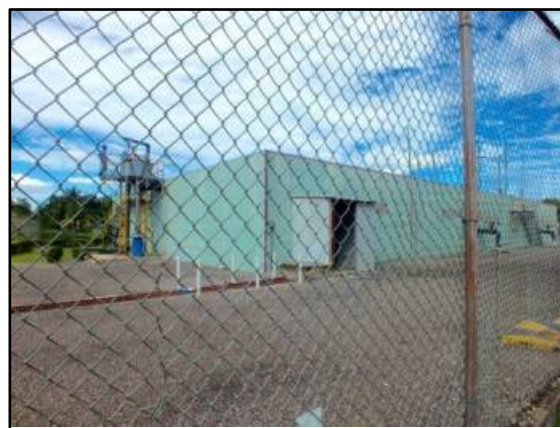
Waste Water Plant
