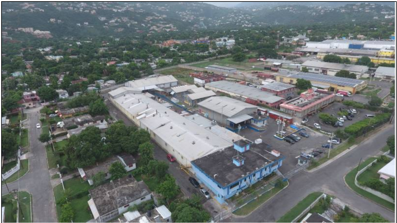
View north of the factory
