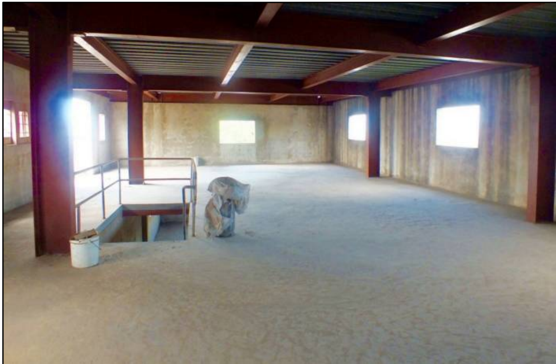
Workshop Building First Floor
