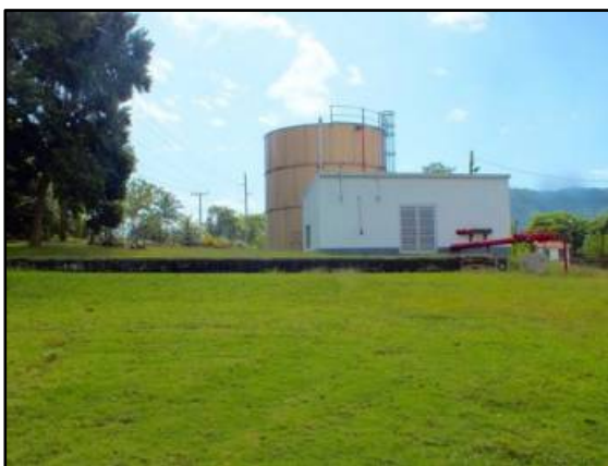
Fire Suppression System
