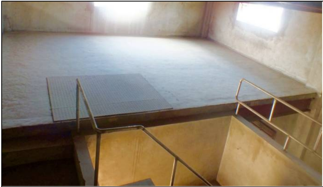
Workshop Building Mezzanine
