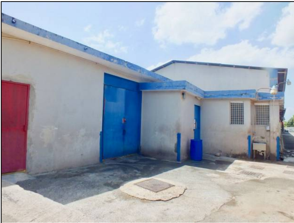
View of the rear of the factory
