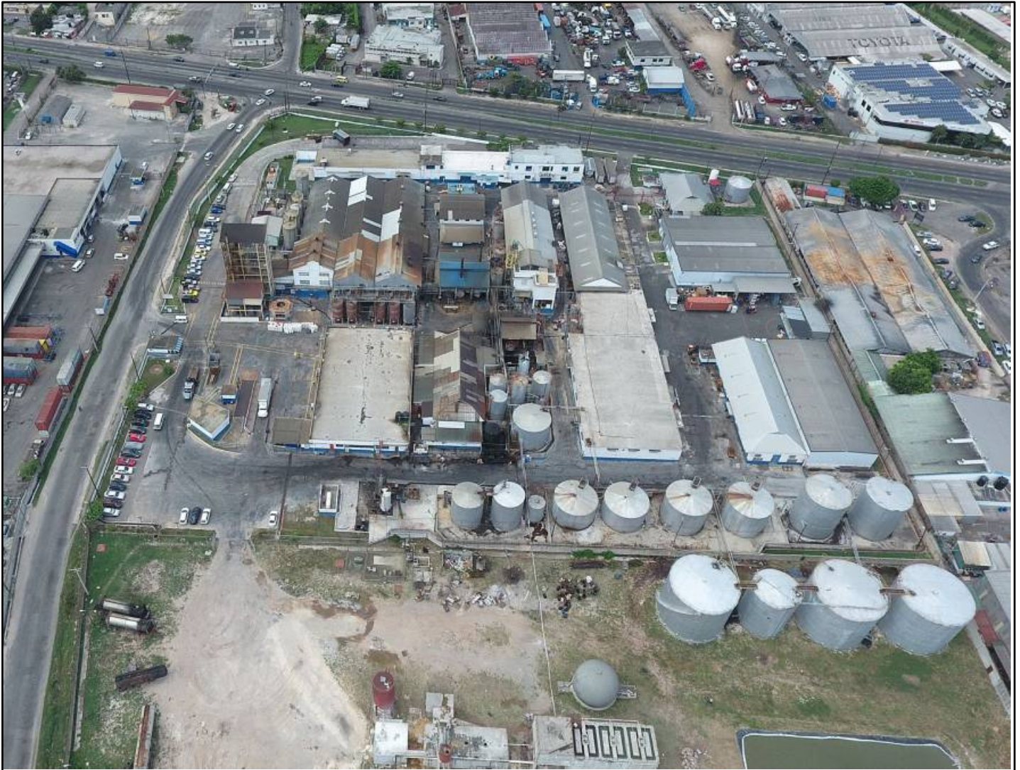
The Factory – view north
