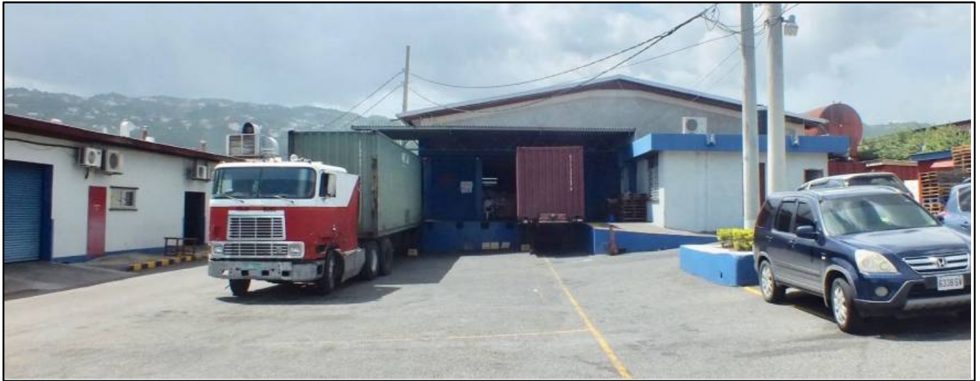
View of finished Goods Warehouse & Training Room
