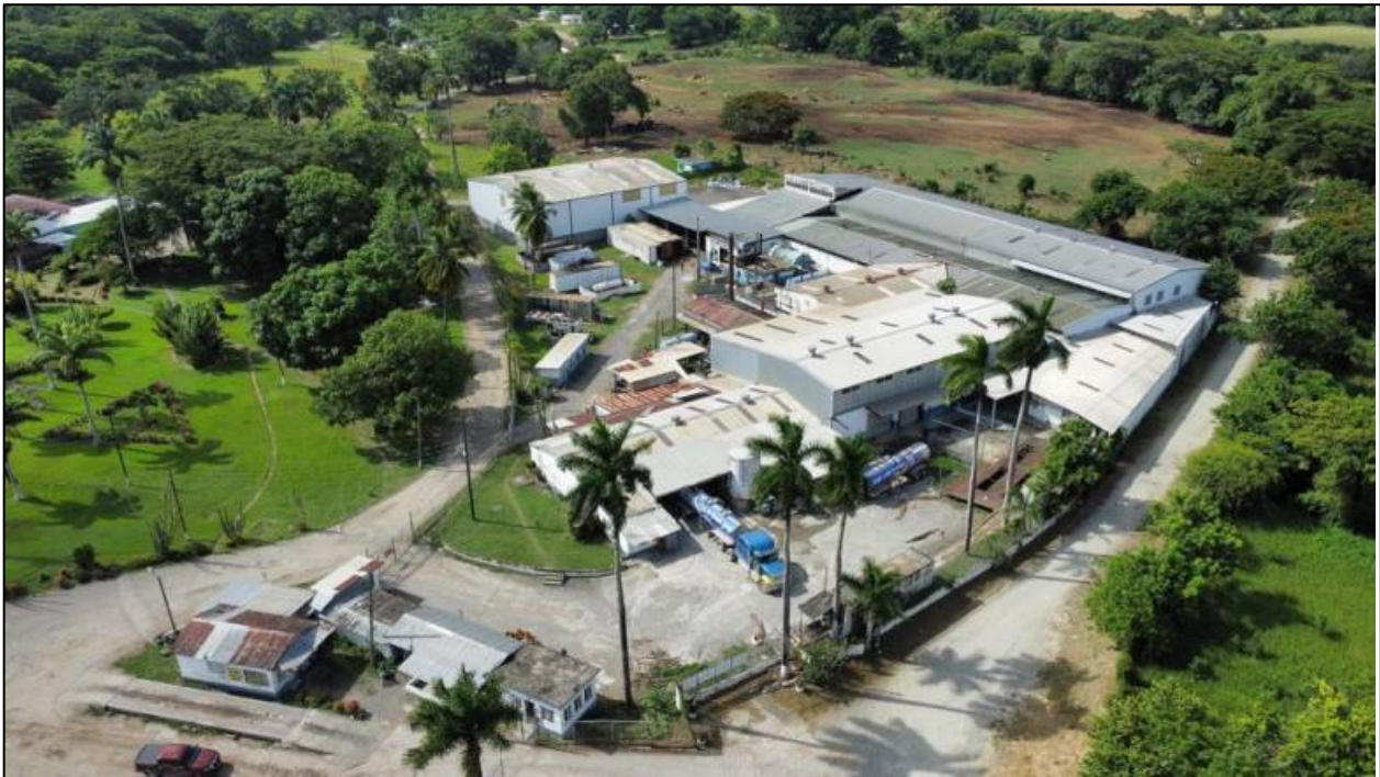
Factory compound July 2023
