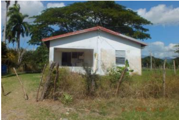
Abandoned Farm Cottage
