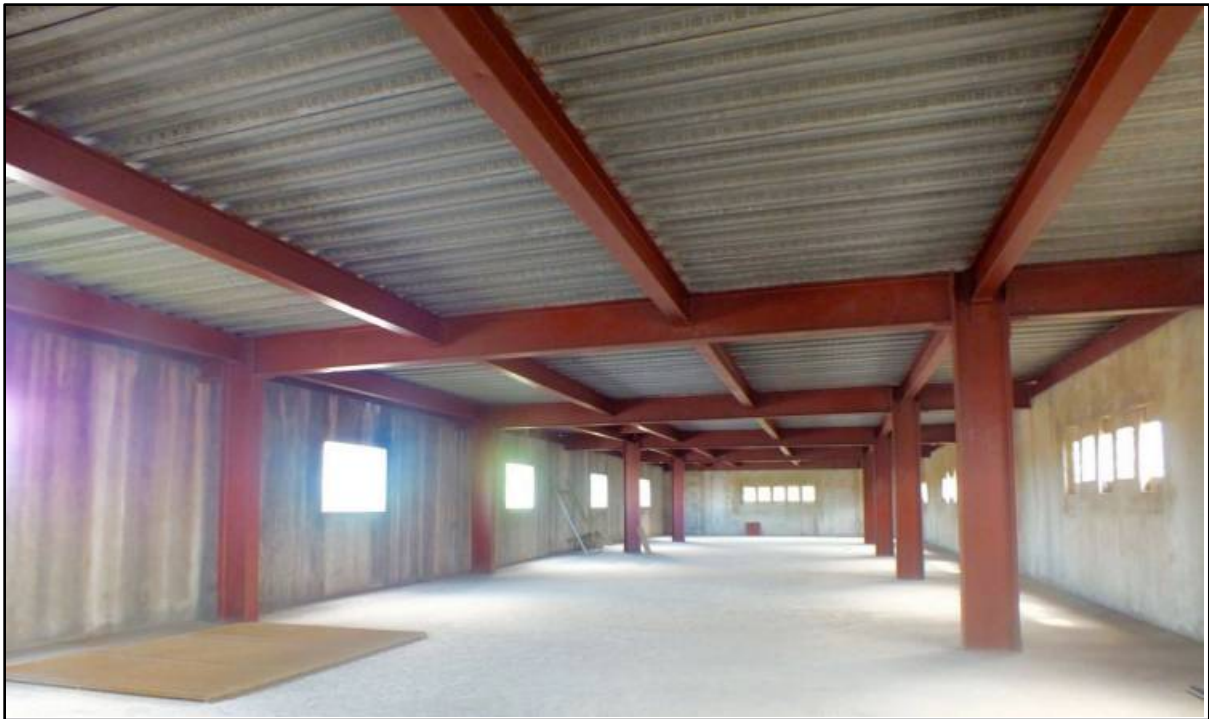
Workshop Building (rear) Ground Floor
