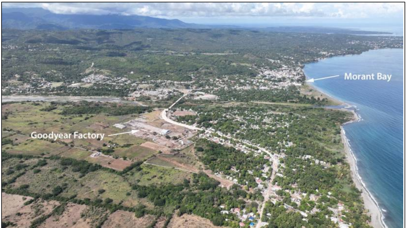
View east showing section for the new Town Center (Goodyear Factory) and Morant Bay
