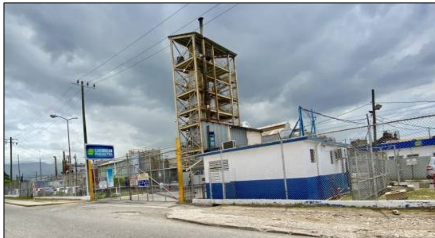
Entrance of property
