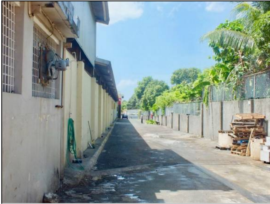
View of the western side of the Factory
