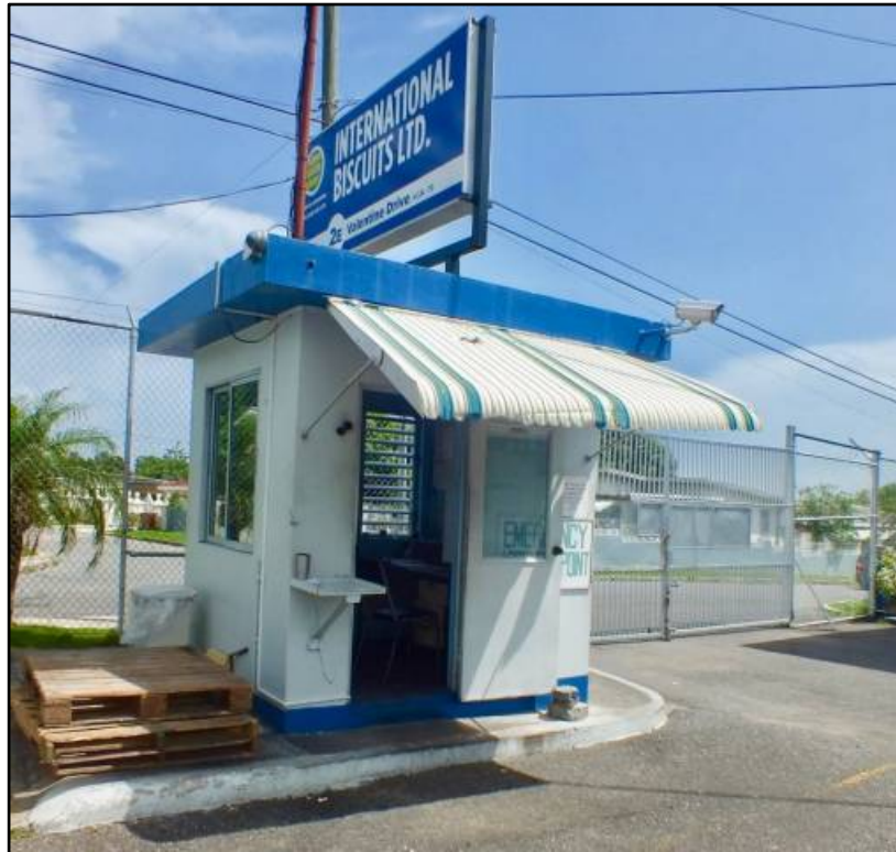
View of Guardhouse & Entrance Gate
