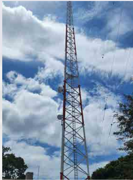
Figure 1 – The new self-supporting tower at Broadcasting House.
