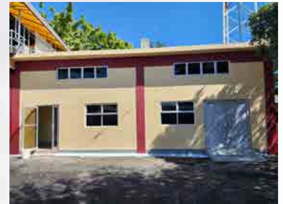
Figure 2 – Newly constructed NOC & DSO equipment room.
