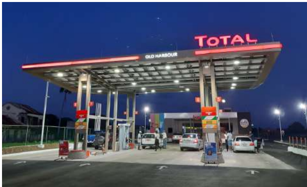
Gas Station at Old Harbour Eastbound On-Ramp
