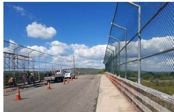
Installation of High Fence at Sharper Lane Bridge
