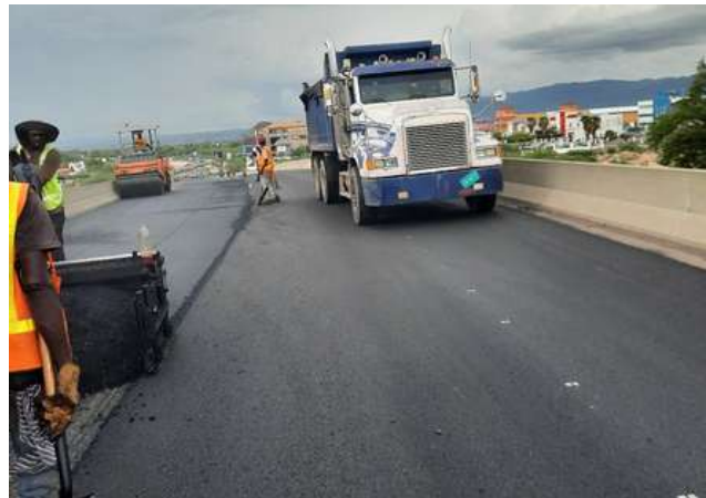
Milling and repaving works along T2 eastbound km6+500 – 5+700
