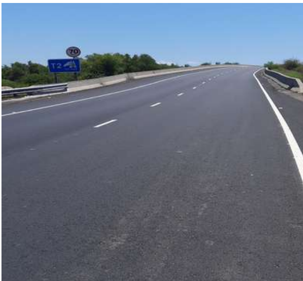
Lane markings at Dawkins Drive Eastbound
