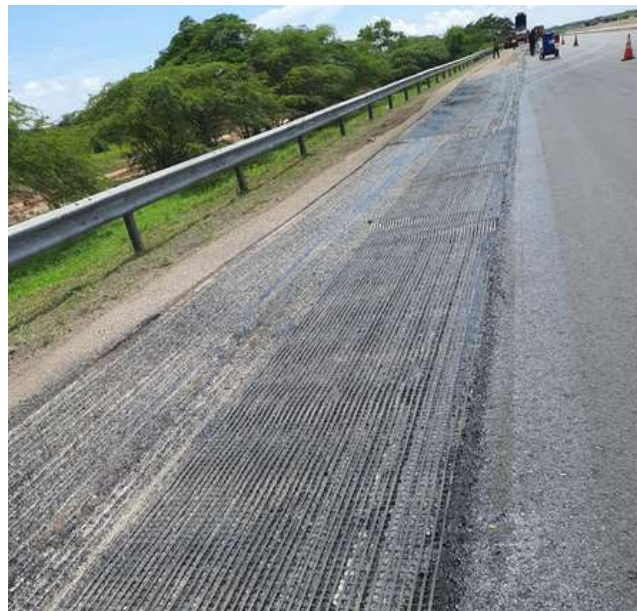
Pavement repairs using geogrid to correct pavement cracks along km16+500 – 17+500
