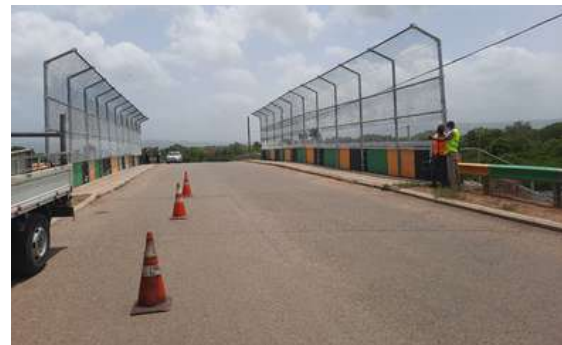
High Fence at Savannah Cross Bridge
