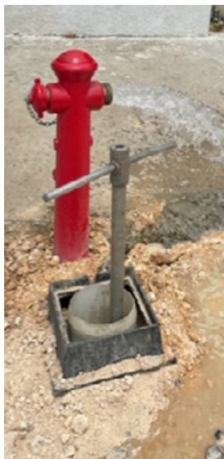
Figure 5a: Testing of the newly installed fire hydrant.
