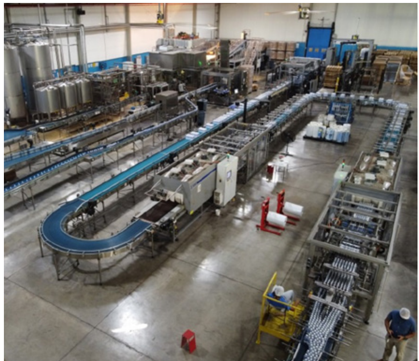
'Wata' plant at Wisynco's Lakes Pen location.
