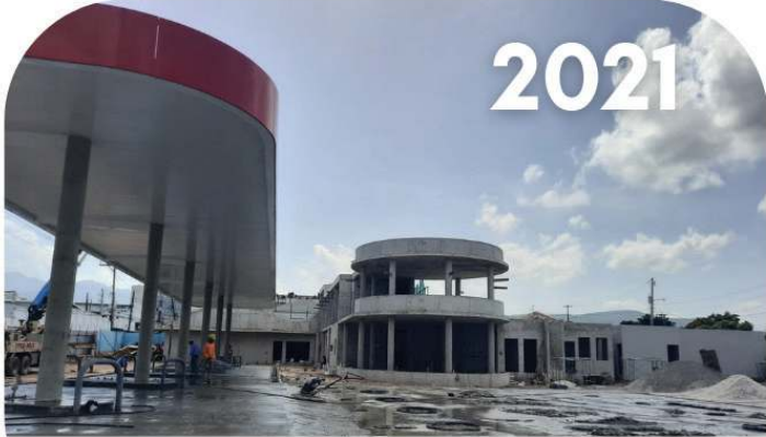
FESCO Beechwood under construction
