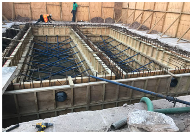
New 22,500 gallon underground water storage tank
