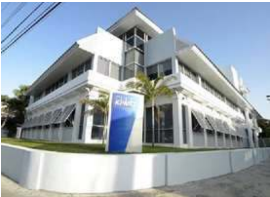
Hastings Office Centre Hastings, Barbados
