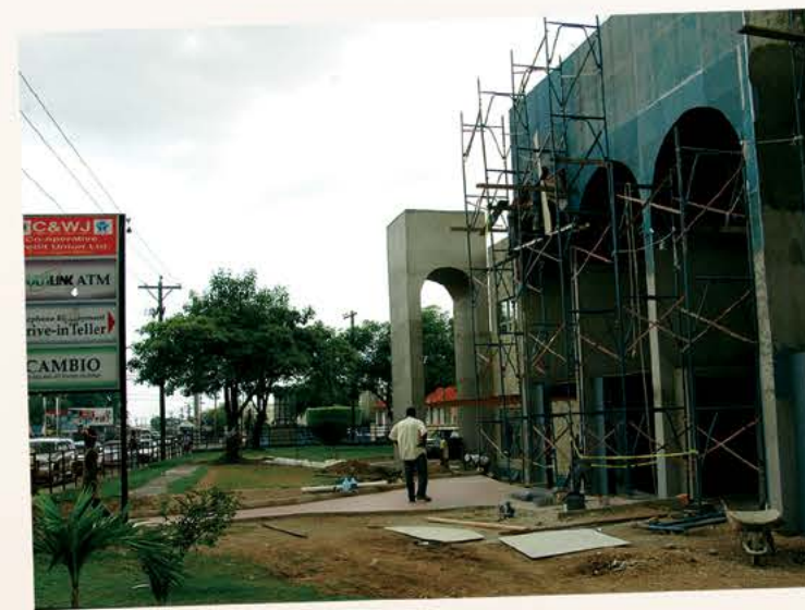
Renovation of Head Office Building (2011)
