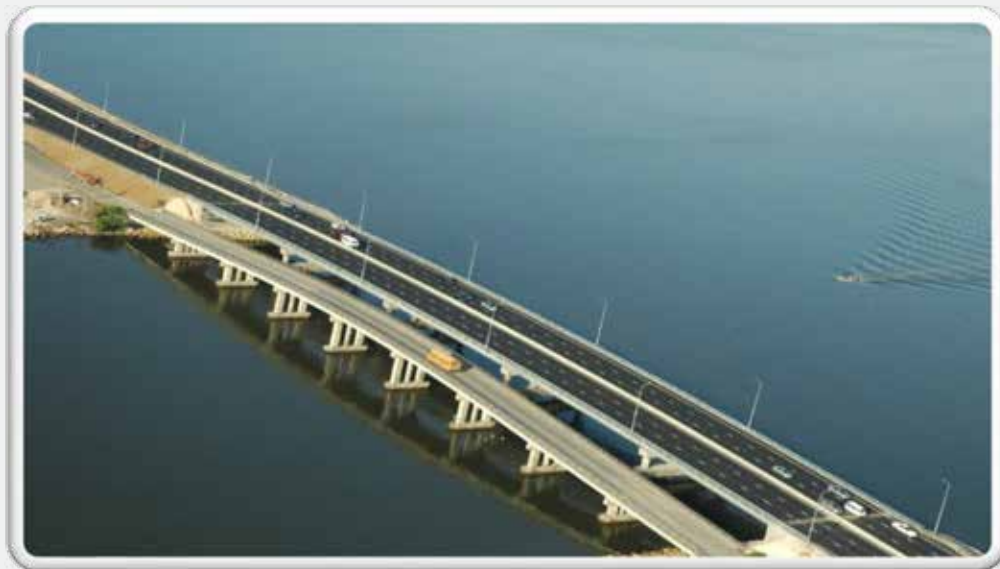
Aerial View of Hunt's Bay Bridge with the abandoned Causeway Bridge in the foreground
