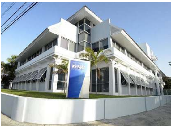
Hastings Office Centre Hastings, Barbados
