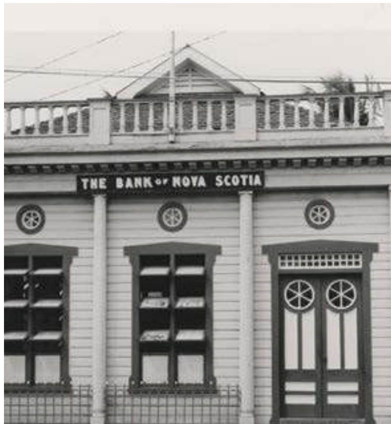
Above (right) – photo of Port Antonio branch exterior from 1960. Courtesy of the Scotiabank Archives.
