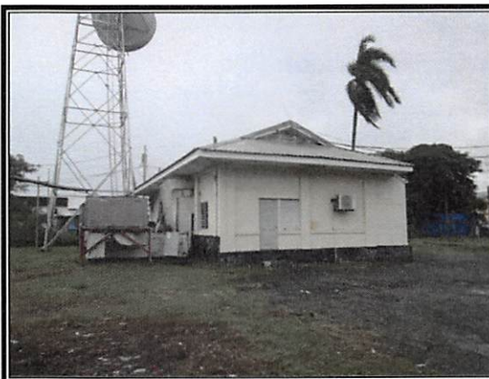
Back of Building #1
