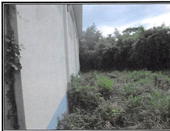
Back of Building #2
