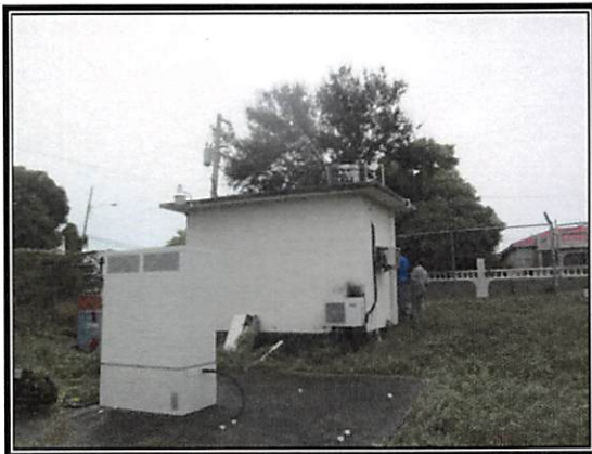
Back of Building
