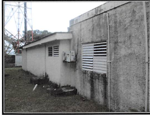
Back of Building #2
