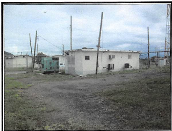
Back of Building #1
