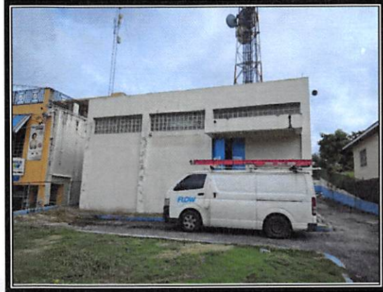
Front of Building
