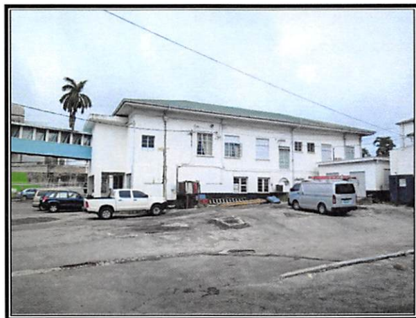
Front Elevation CO building
