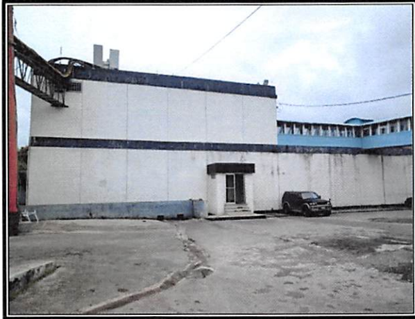
Front Elevation CO building
