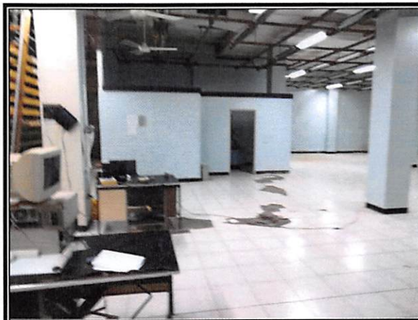
Internal CO building
