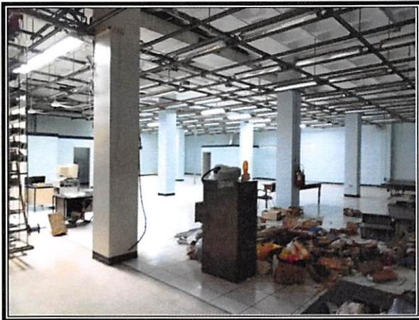
Interior CO building
