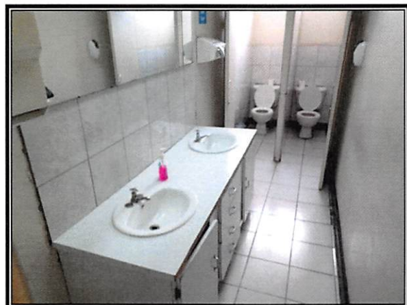
Bathroom – Office building
