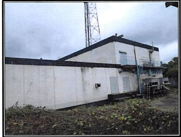
Rear Elevation CO building
