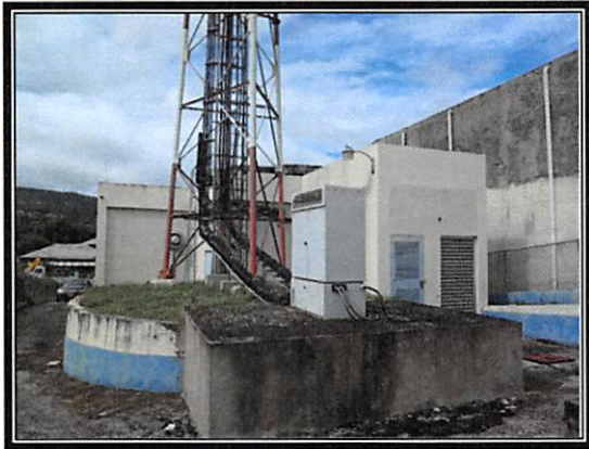
Back of Building
