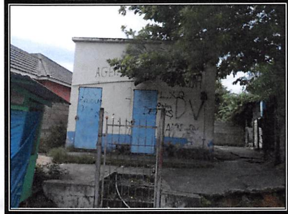
Front of Building
