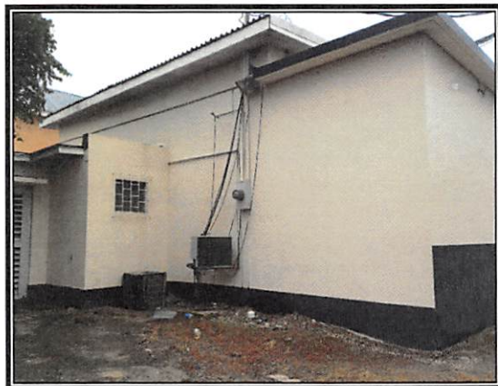
Back of Building
