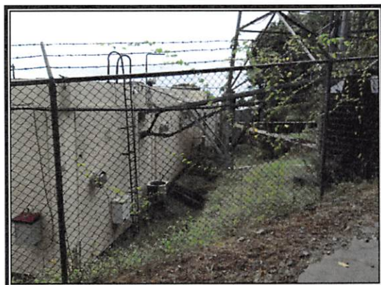
Back of Building 1.
