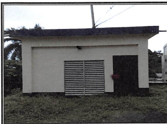
Front of Building 2.
