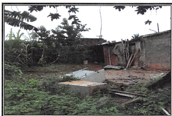
Back of building
