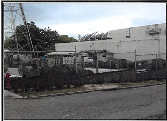
Back of Building
