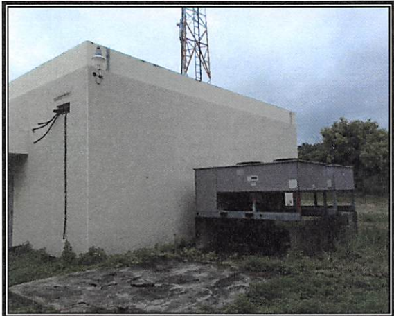
Back of Building 1
