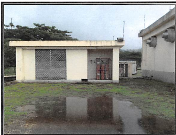
Front of generator building
