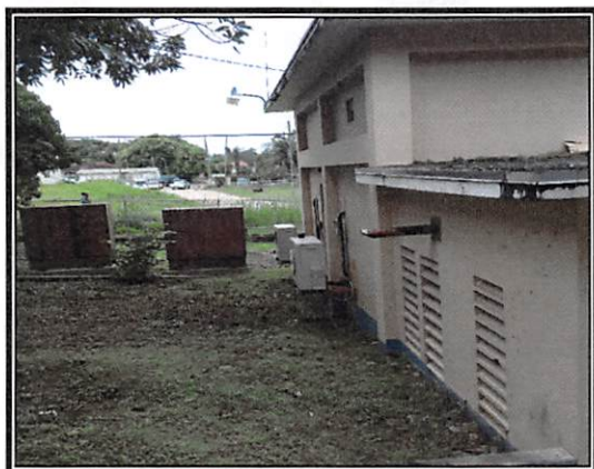
Back of Building
