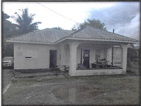
Front View Building #2
