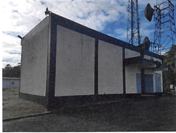
Front of server Building
