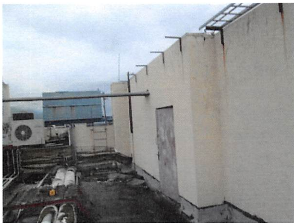
Roof of Main Building
