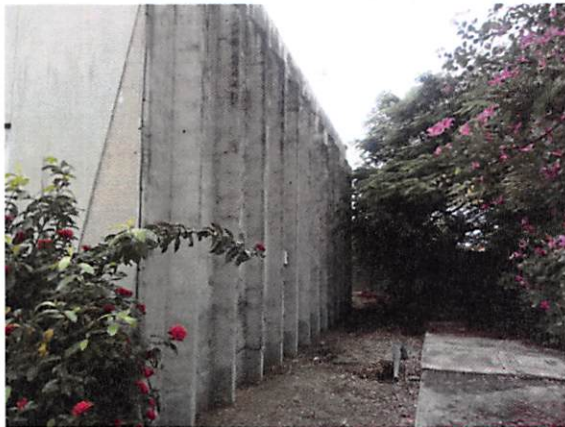
Back of Building
