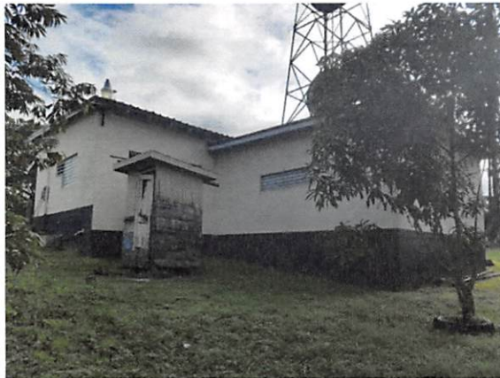
Back of server Building
