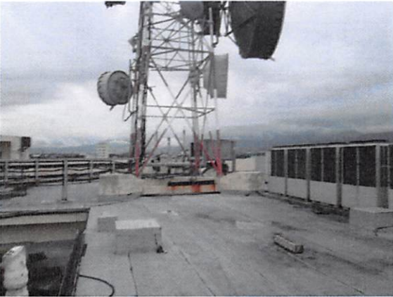
Roof of Main Building
