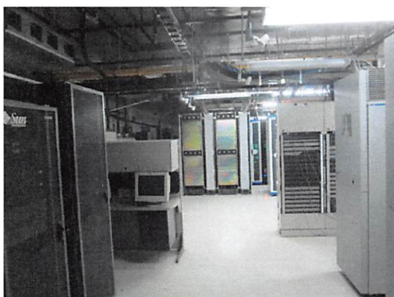
Main Building - Interior
