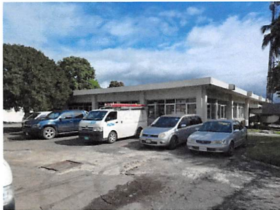
Side & rear of Building
