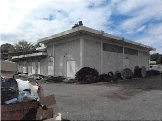
Side & rear of Building
