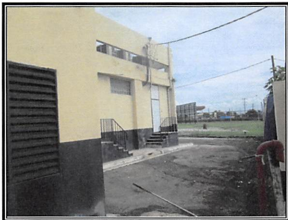
Back of Building 1
