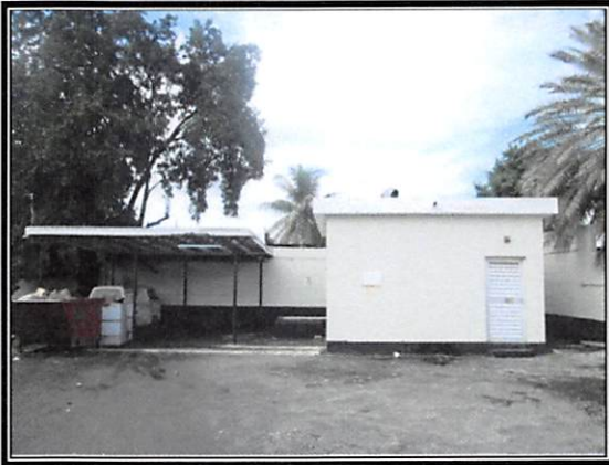
Parking Shed and Generator Buildings
