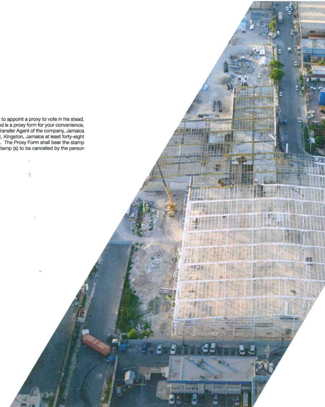
Aerial view of the KWL Total Logistics Facility construction site.
