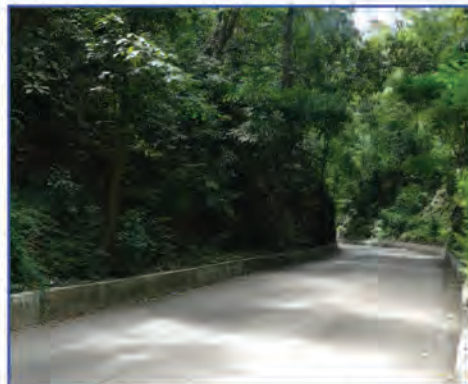
Concrete Road in Fern Gully, St. Ann
