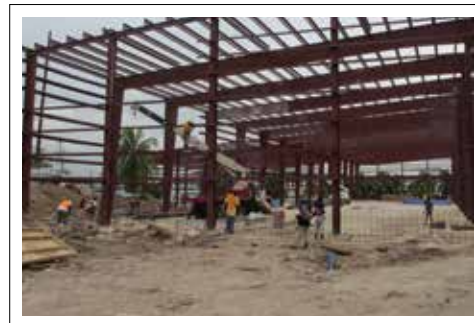
Manufacturing Plant building under construction at White Marl, St. Catherine.
