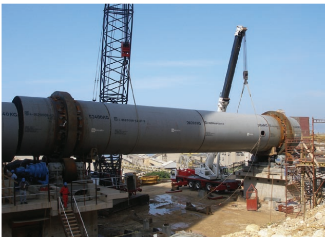
Rotary kiln: two central kiln sections were joined and then lifted together by two cranes to connect to the tyre support sections that are already in place.
