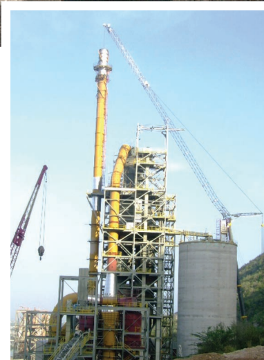
Preheater tower: the last section of the flue gas stack being installed. It was designed based on Environmental Air Dispersion Models.
