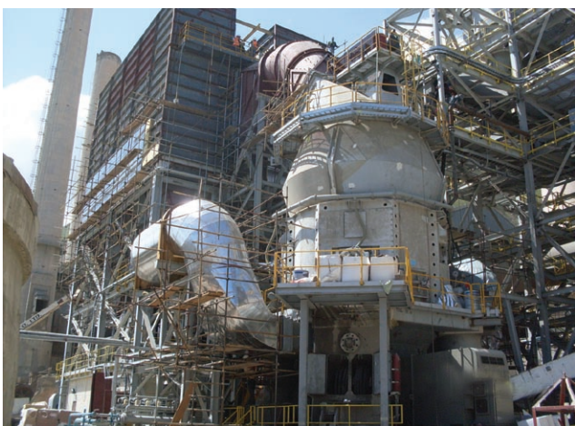
Cement mill no.5: sections of the vertical roller mill equipment are being tested while process gas ducts and the mill vent baghouse are being insulated.
