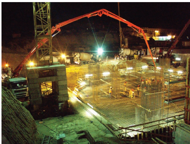
Preheater tower foundation: concrete pour for the preheater tower foundation in progress. Overall volume was in excess of 1800 m 3 using Carib Cement Plus.
