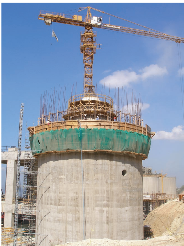
Homogenising silo: continuous slip forming of the 7000 t homogenising silo in progress for 21 days. Visible is the internal silo cone for raw meal extraction.
