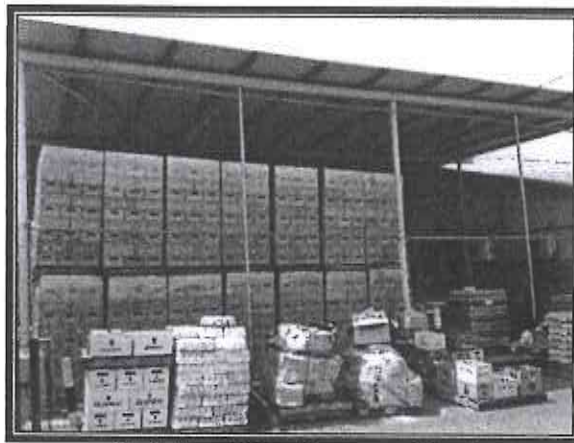
Building III – Storage Shed
