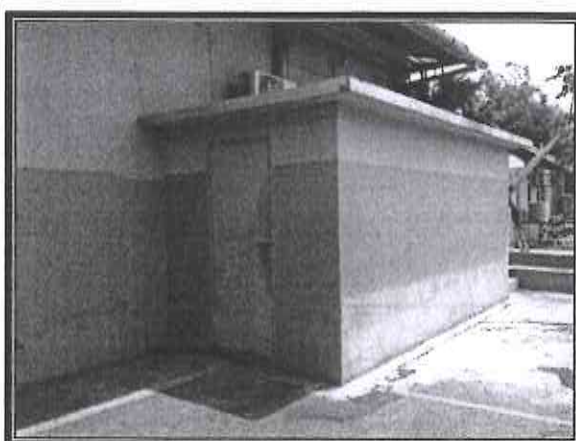
View of the computer server room
